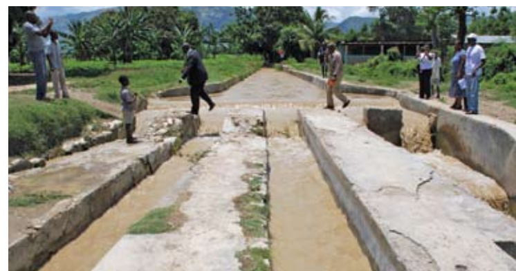
Water intake system that feeds the irrigation canals of Plaine du Cul de Sac.
